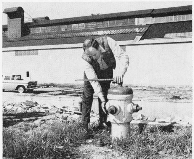
Readiness is the key point in fire control. Everything must work right in a fire emergency. So, it's 'round and 'round every day to some piece of equipment to be sure it is ready. Here, it's just a 'hydrant' but very important. "Red" makes sure it has not been damaged, isn't leaking, can be opened, and is ready to go.
